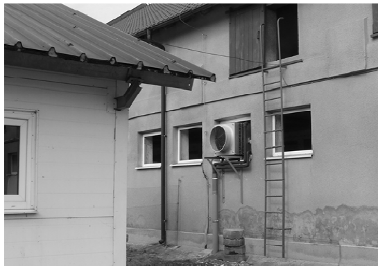
Figure 2. Part of the renewable energy laboratory and cowshed with the fan coil unit.
